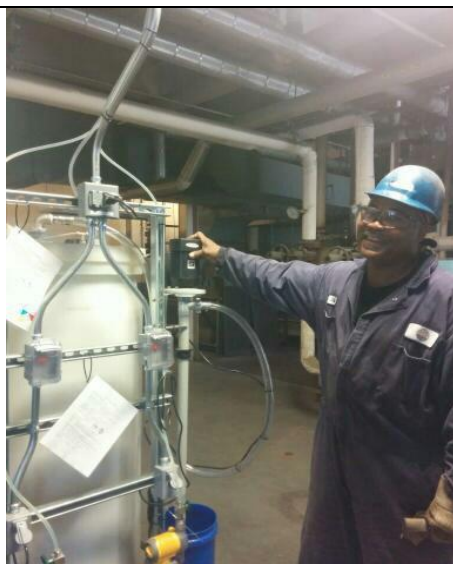
Figure 29 Technician checking the installation of chemical injection to fly ash
